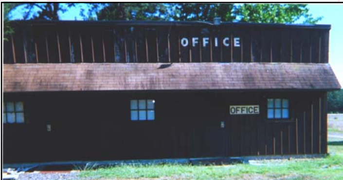
BEFORE Front of Office Building
